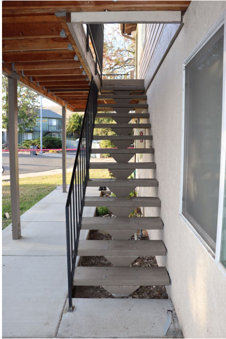
Figure 3. Stairwell leading to upstairs landing and Units D and A.
