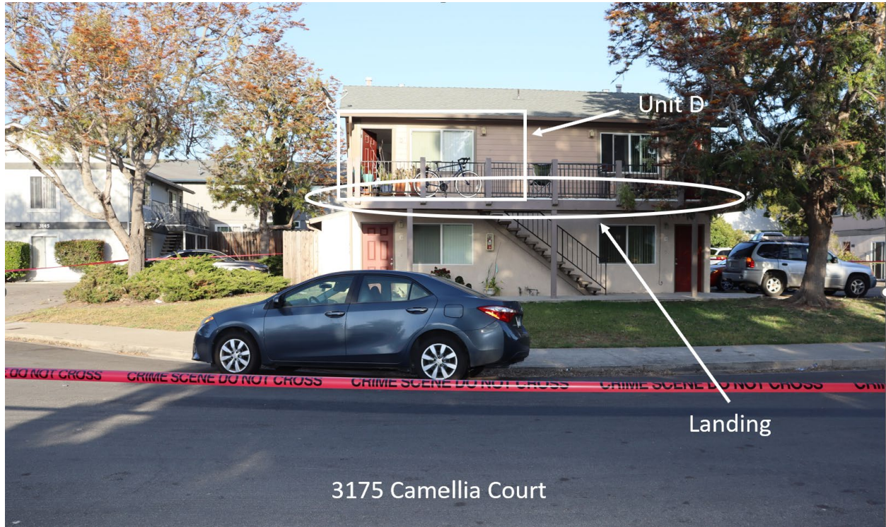
Figure 1. 3175 Camellia Court, depicting Unit D, second story landing, and stairwell.
