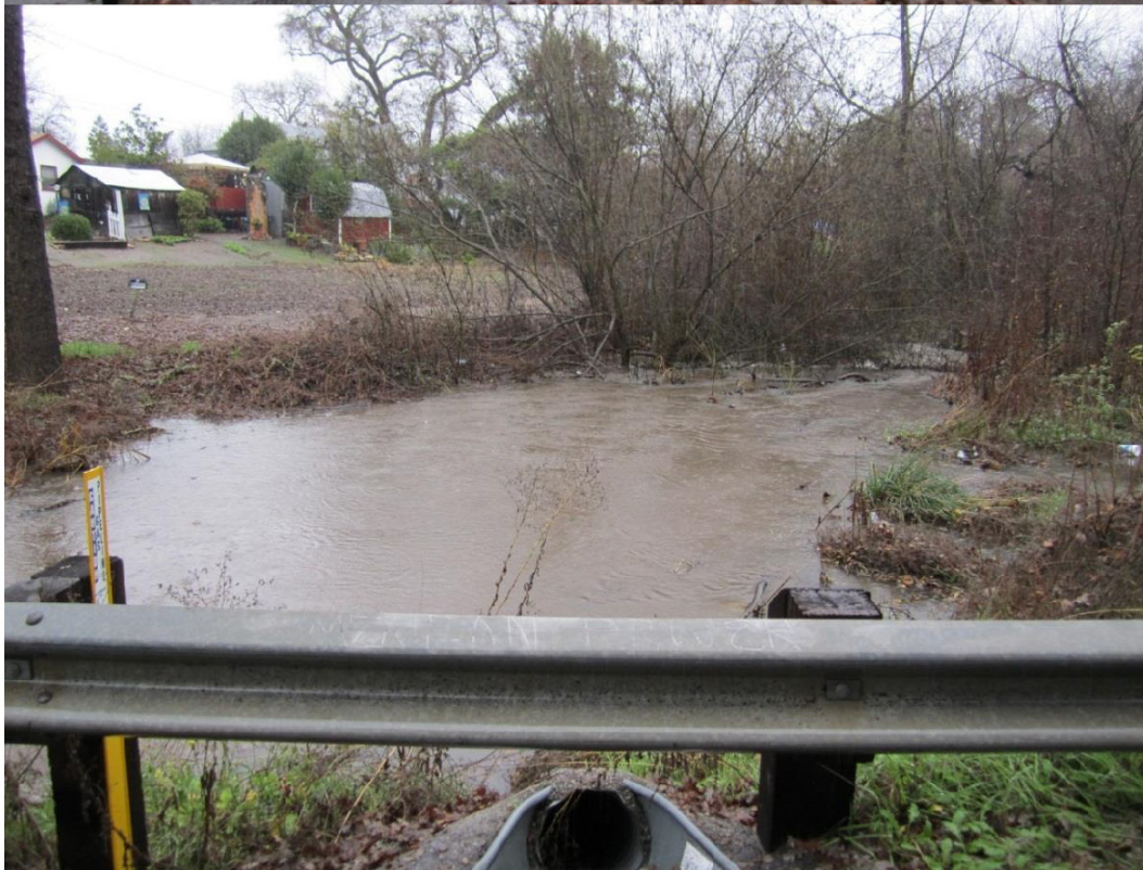
Bridge at Florence Street
