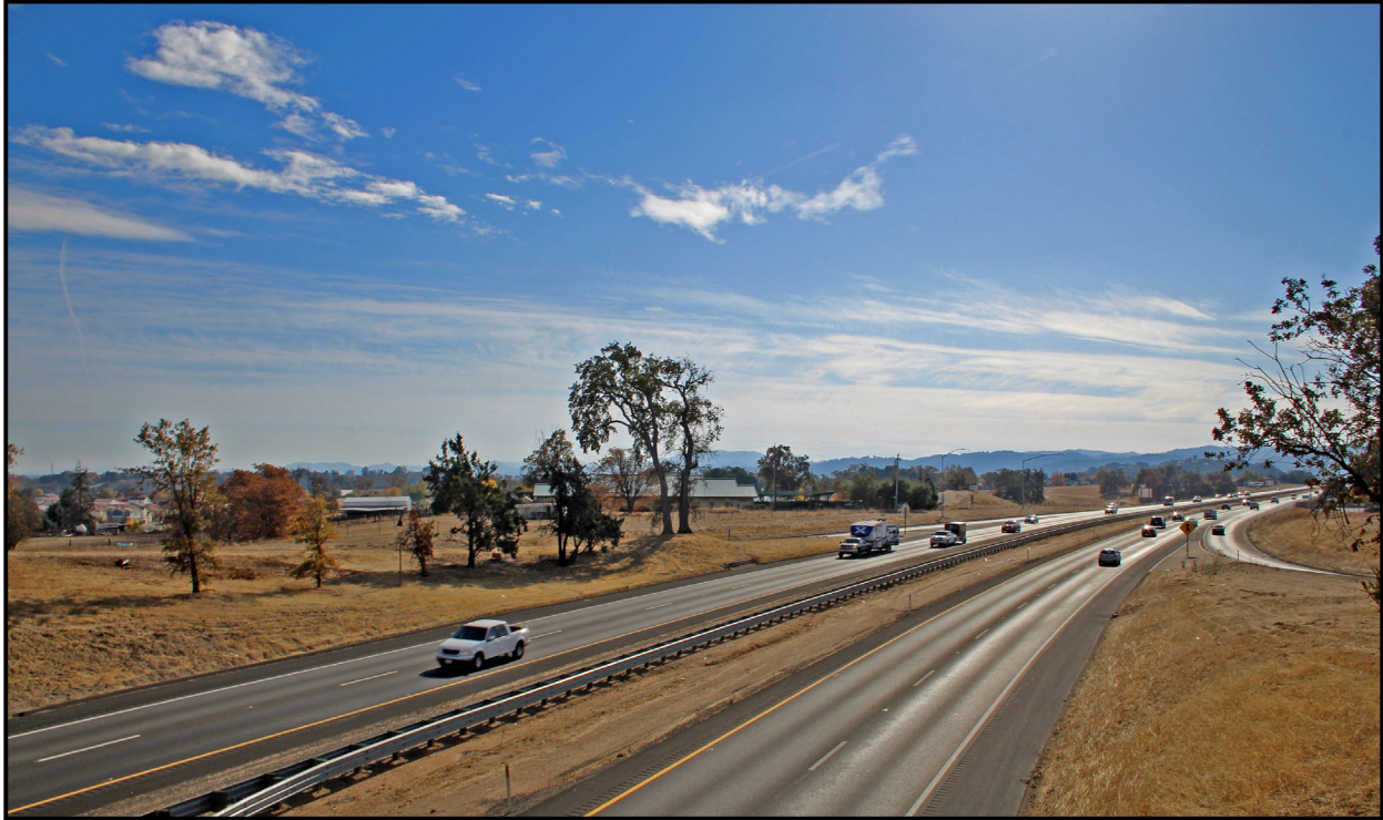
(a) Existing view.
