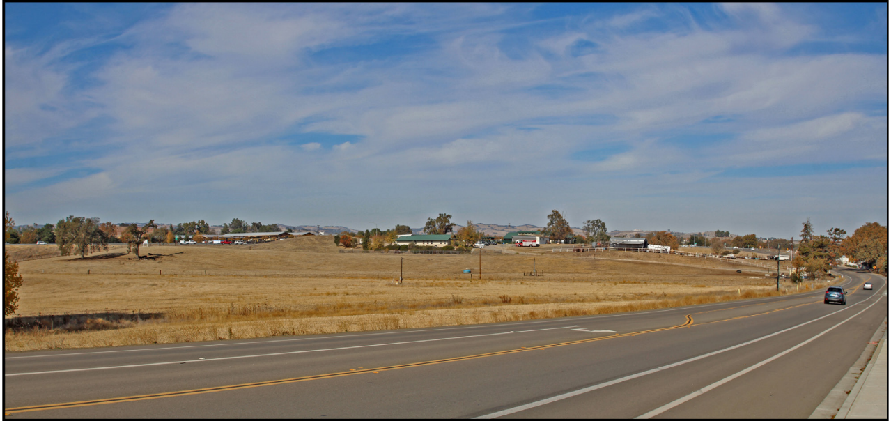
(a) Existing view.
