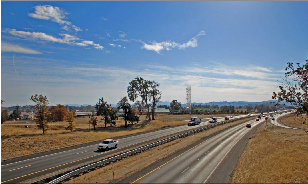
Figure 12. Key Viewing Area 3: Photo-simulation of the project from the Main Street overcrossing looking south.
