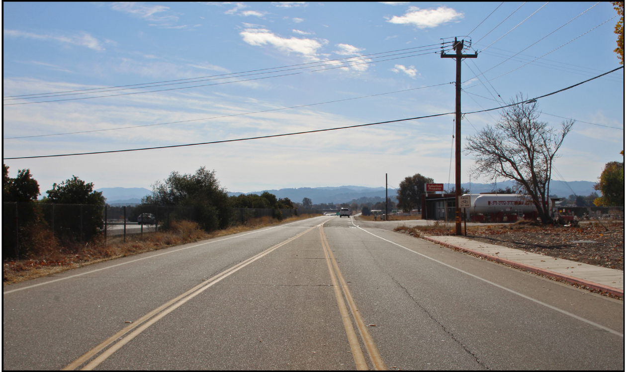
(a) Existing view.
