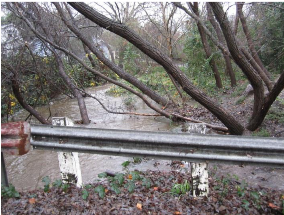
Salinas Ave. Bridge at Eddy Street
