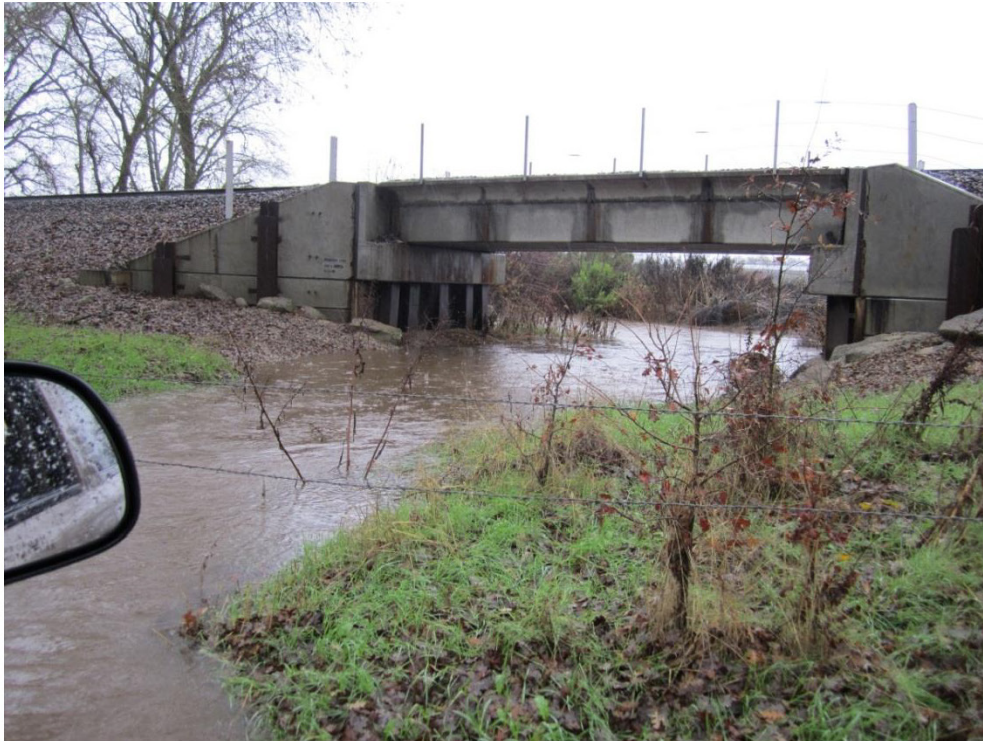
East side of Train Bridge
